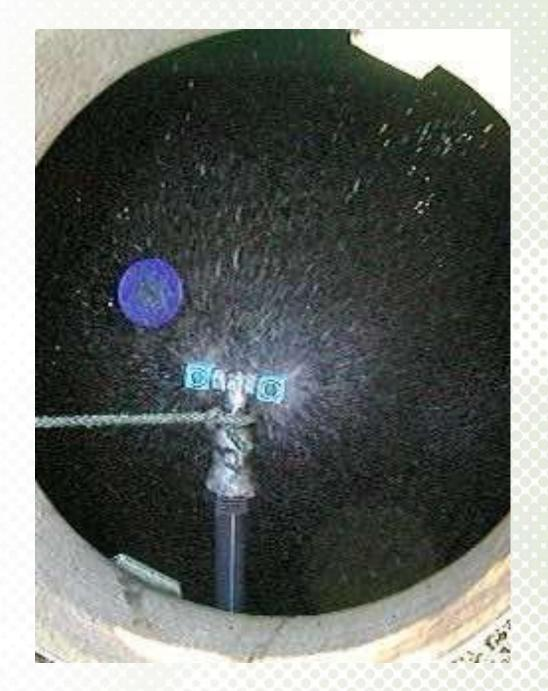
Biofilter: trickling filter (fixed biofilm)
